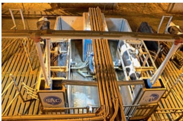
Each of the SAC Futureline robots serves two boxes. Cows enter from the cubicles at the rear (top of the picture) ...
