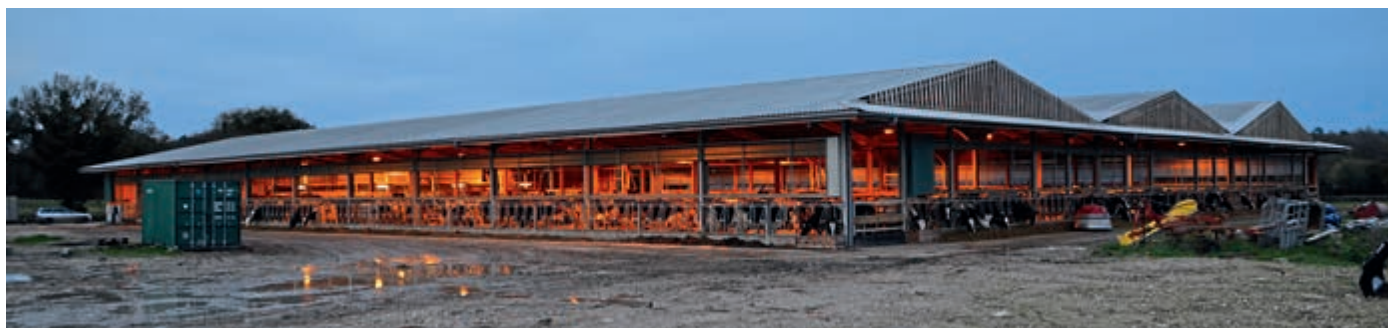
Without feed passages splitting the housing area, yoke barriers form three sides of the building to provide enough feed space for over 400 cows.
