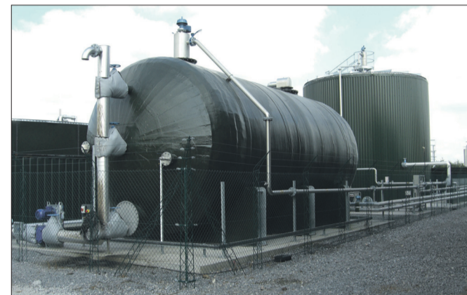
The 'plug and play' anaerobic digester can be installed in about three weeks, at a quarter of the cost of a traditional AD system.
