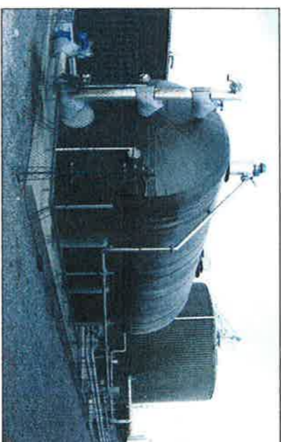
The 'plug and play' anaerobic digester can be installed in about three weeks, at a quarter of the cost of a traditional AD system.
