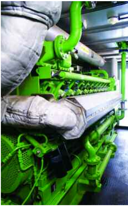
The biogas is fed to two huge V20 engines that generate enough electricity for 4600 homes.
