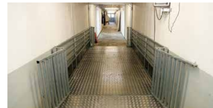
An easy-loading system allows lorry drivers to load pigs without a staff member present.
